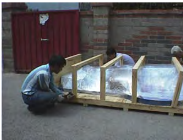
3. Fix the supporting frames.
